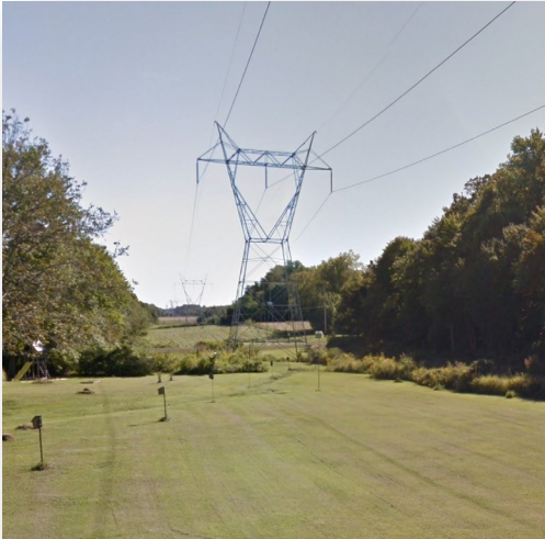
Existing 230 kV corridor
