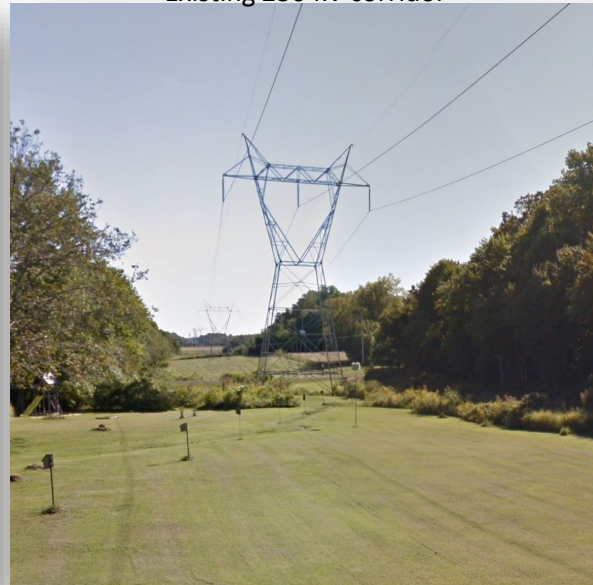
Existing 230 kV corridor
